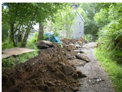
The trench from the water meter
