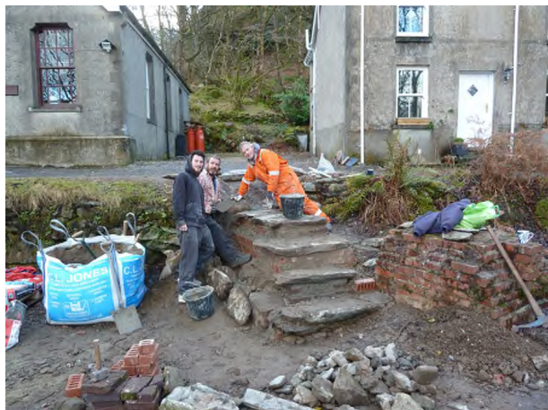
Building the new car park steps
