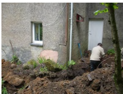
and the pipe laid
